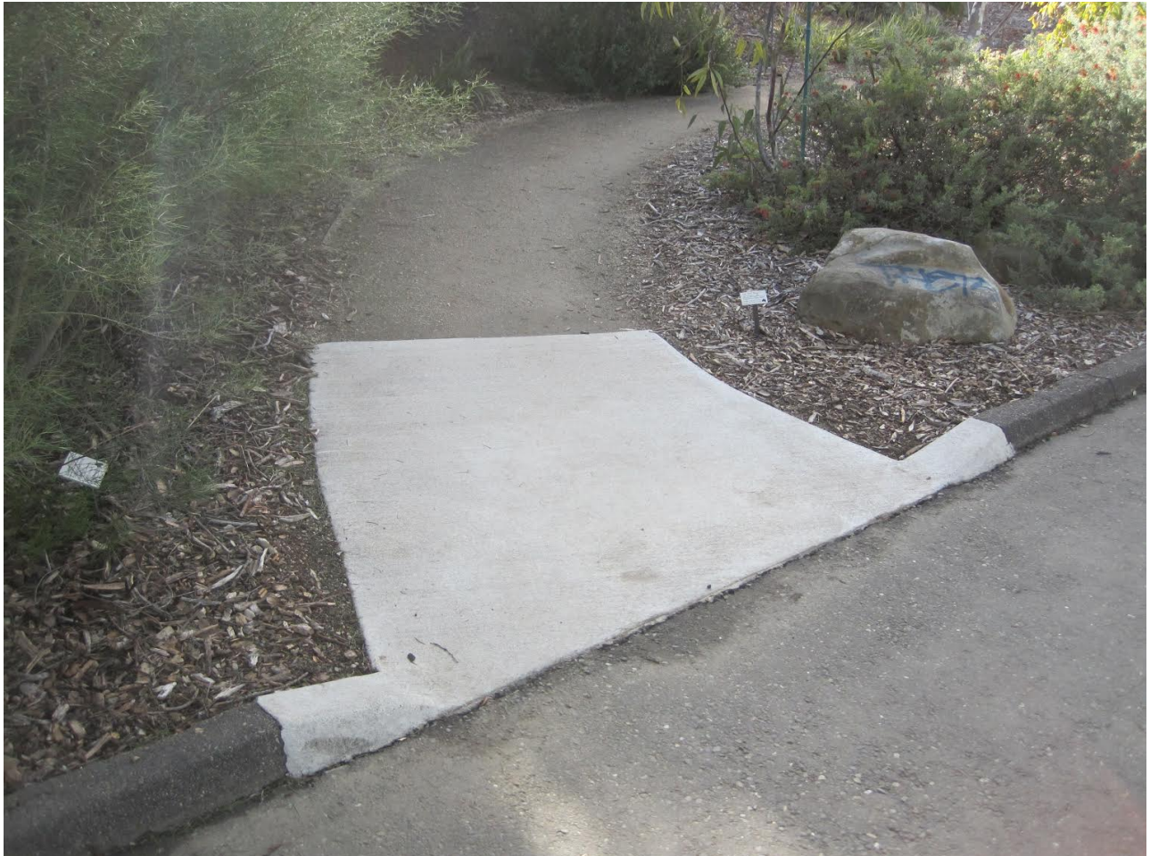
Example of a ramp transitioning the asphalt path to decomposed granite with poured concrete
